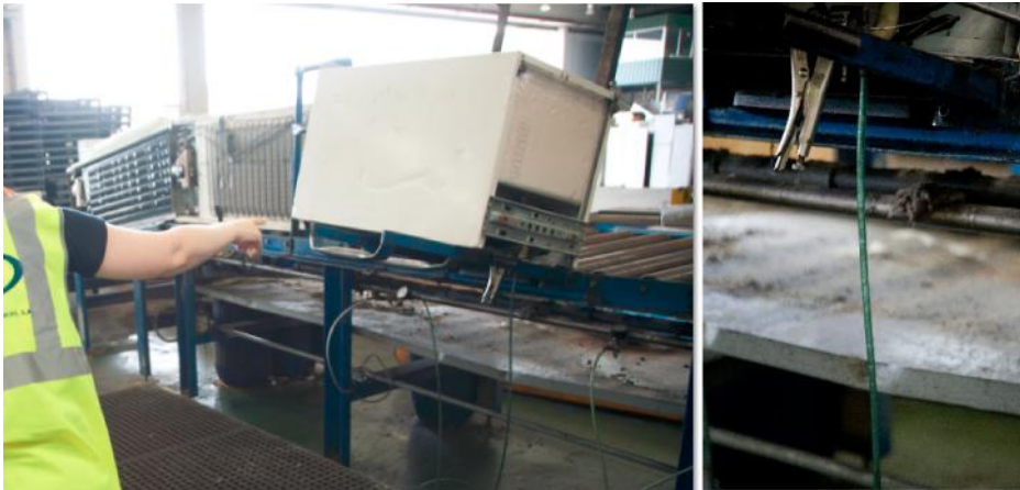
Picture 5. Left: removal of oil and gas from the cooling circuit. Right: detail of the removal of oil and gas from the cooling circuit.
